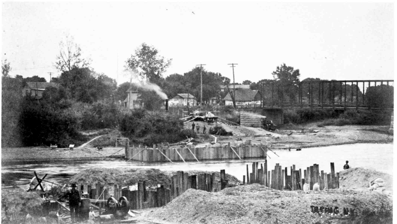
Buffalo & Erie Trolley Bridge, under construction at Irving about 1908.
